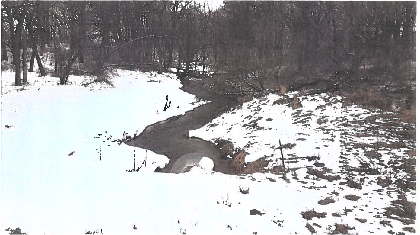
Existing CMP – Looking Upstream
